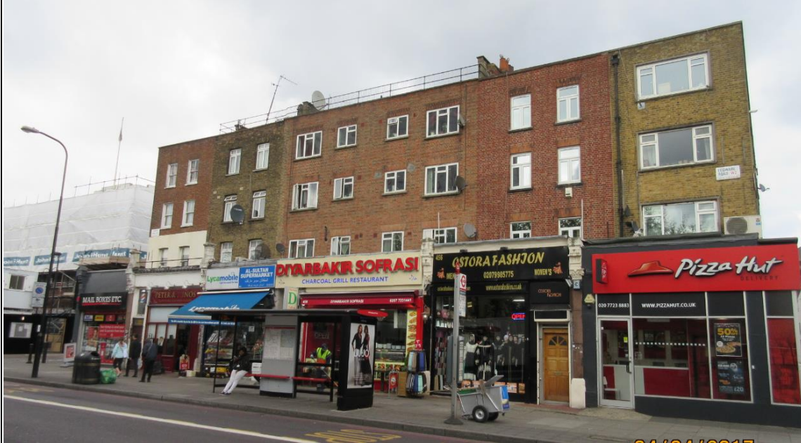
Edgware Road frontage
